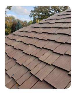
DaVinci Roofscapes mimick wooden shake shingles, yet they are made of a fireresisitant composite material. *Photo Credit:* RoofingContractor.com
