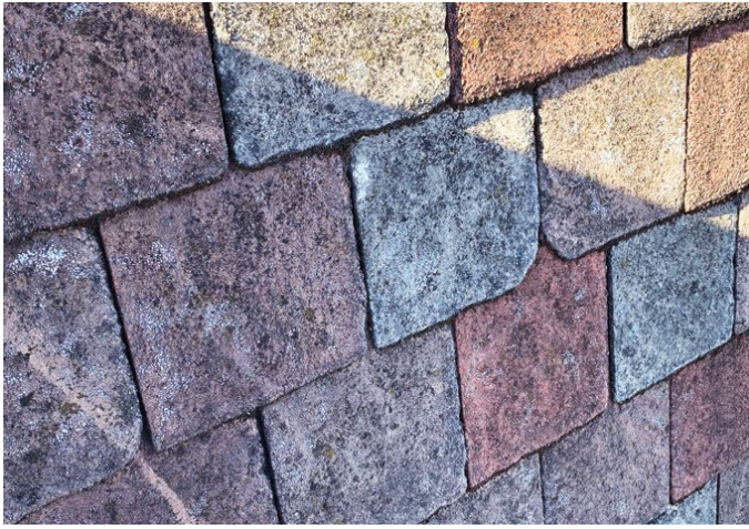
Figure 5. (Left) Asbestos shingles were often used as a substitute for traditional slate roof shingles. The historic asbestos roof on this rehabilitation project had reached the end of its lifespan and required complete replacement. (Right) Given the limited replacement materials available to match the historic asbestos shingles, utilizing natural slate was determined to be the best visual match for the original shingles and design intent in this instance. Photos: Crosskey Architects.
