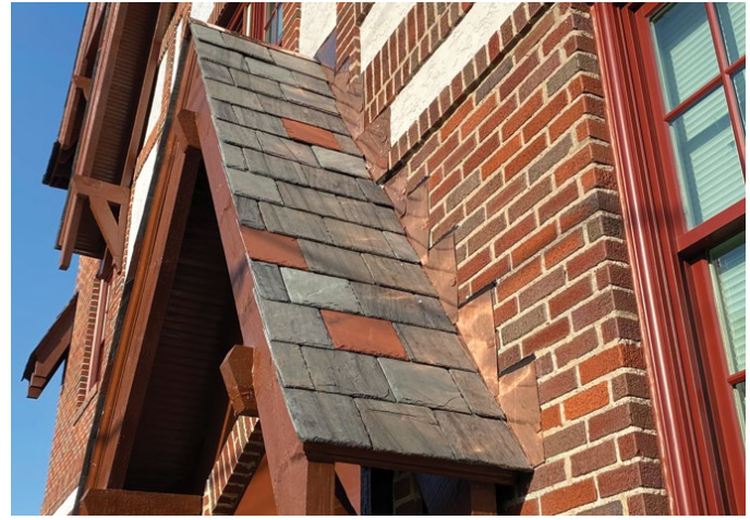
Figure 5. (Left) Asbestos shingles were often used as a substitute for traditional slate roof shingles. The historic asbestos roof on this rehabilitation project had reached the end of its lifespan and required complete replacement. (Right) Given the limited replacement materials available to match the historic asbestos shingles, utilizing natural slate was determined to be the best visual match for the original shingles and design intent in this instance. Photos: Crosskey Architects.
