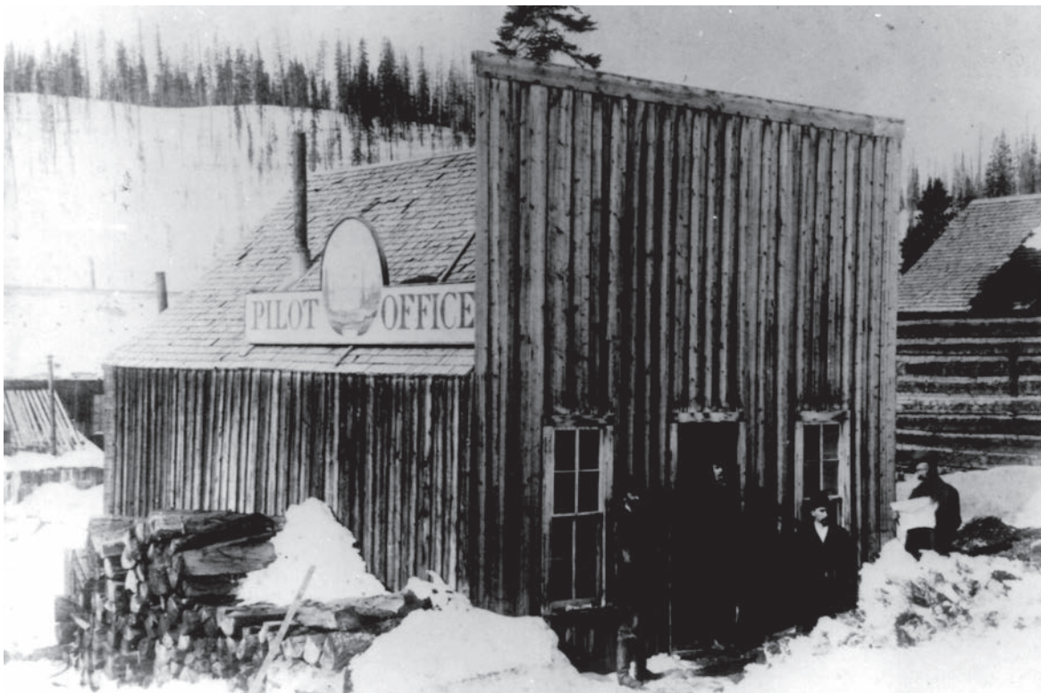
The Pilot Office in its early years exhibited the simple false fronts of the vernacular commercial architecture of Crested Butte. The vertical board wall screened a typical gable roof.
