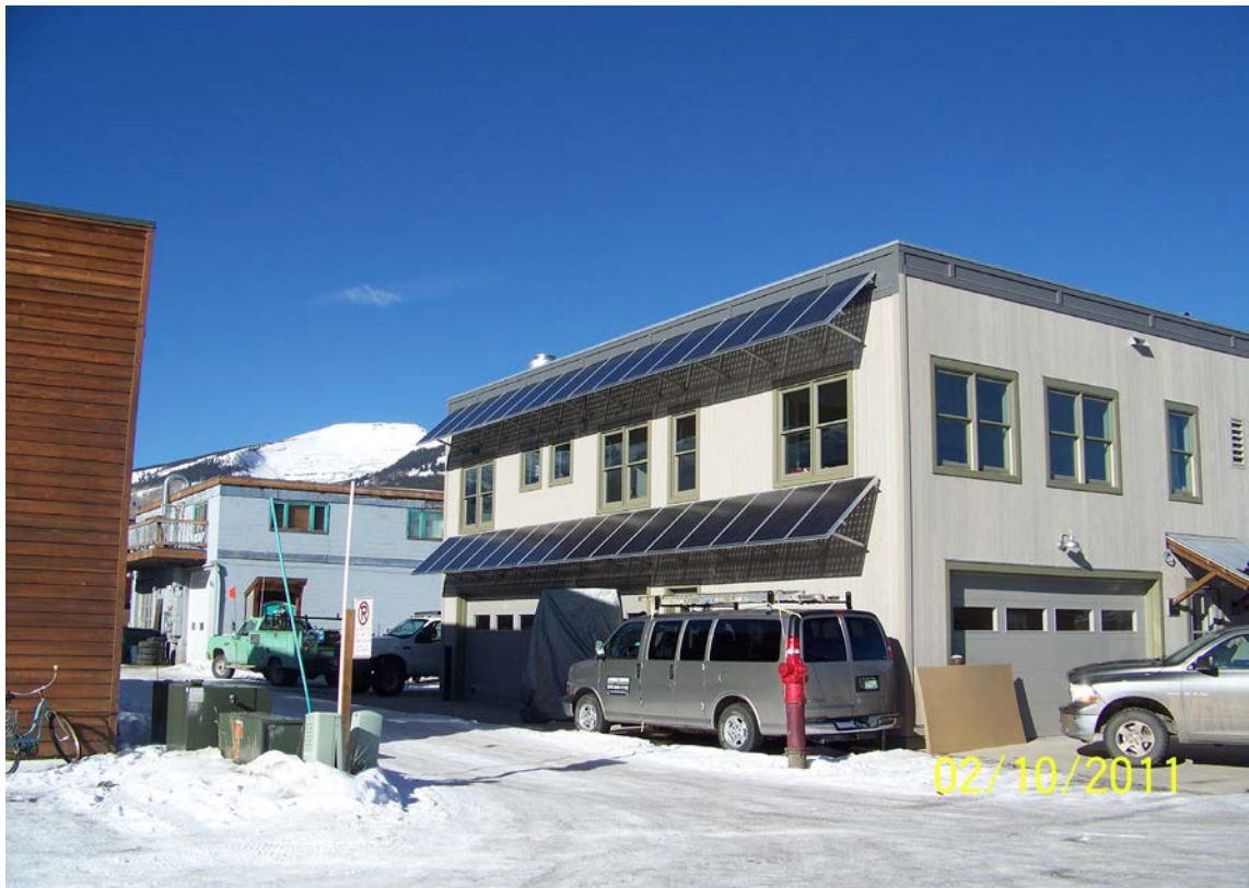
The awning solar array attached to the rear of 330 Bellevue is an effective method to increase the energy production or off-set ground surface heating.
