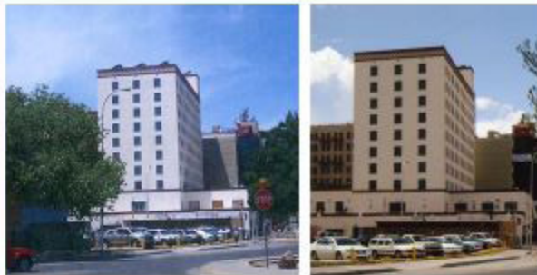
Left, solar panels create a new sawtooth feature on the roof of a historic hotel. Right, after lowering the angle of the panels, they are no longer visible from this vantage point.
