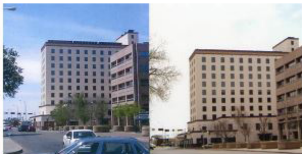
The original angle of the solar panels (left) was lowered (right) to maintain the prominence of the roofline and cornice. Only the very top of the panels can still be seen.
