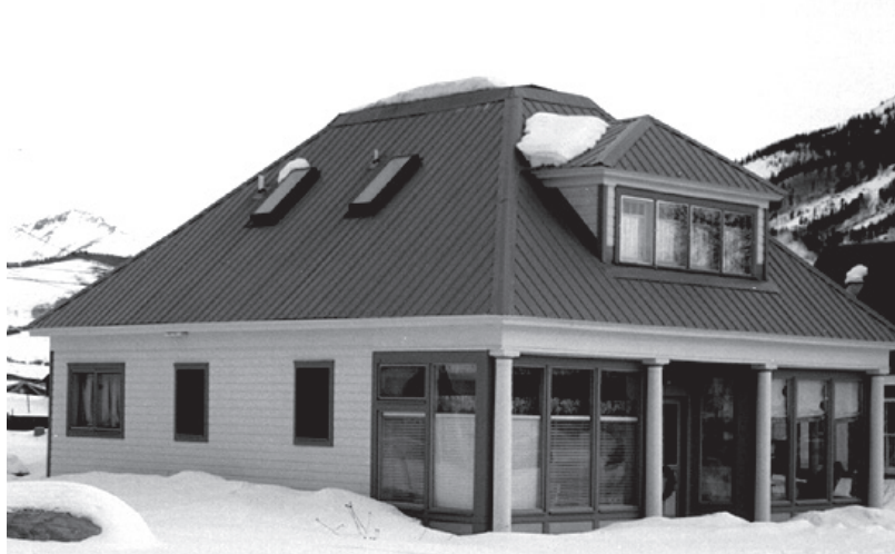
The hipped-roof house is characterized by the pyramidal shape of its roof.
