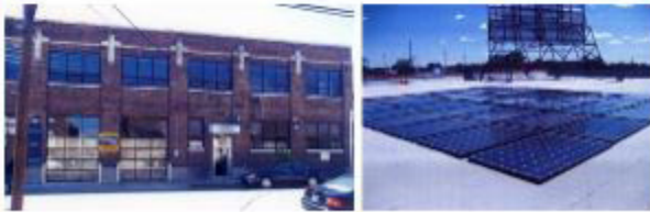
This "invisible" installation of solar panels on a historic industrial building—hidden behind a low parapet—meets the Standards for Rehabilitation.
