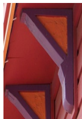
Historic corbel detail Simplified modern corbel detail
