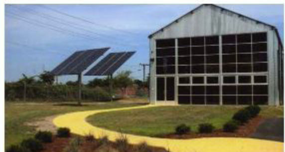
Pole-mounted solar arrays can be appropriate alternatives to rooftop installations such as on this industrial site.
