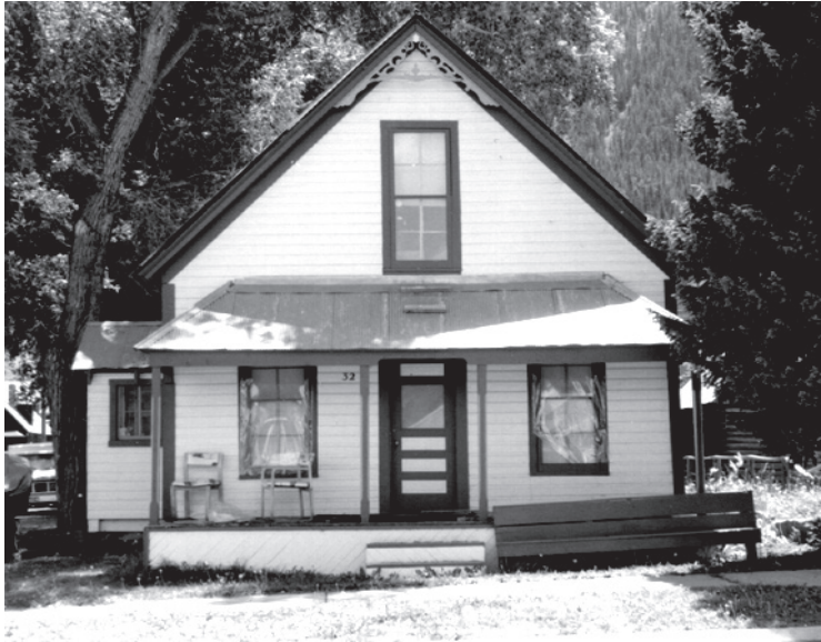
The gable-end house roof ridge is usually perpendicular to the street.
