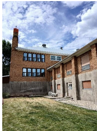
Rear (north) new windows installed and parge coat repairs
