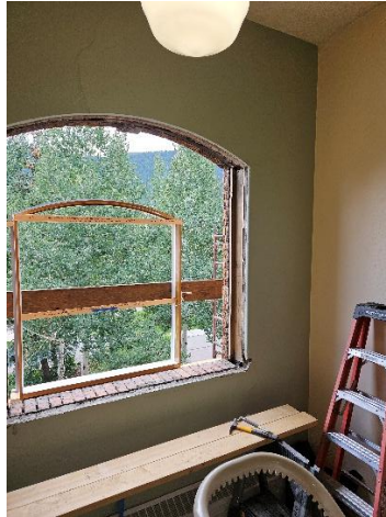
Front (south) arched window frame installation
