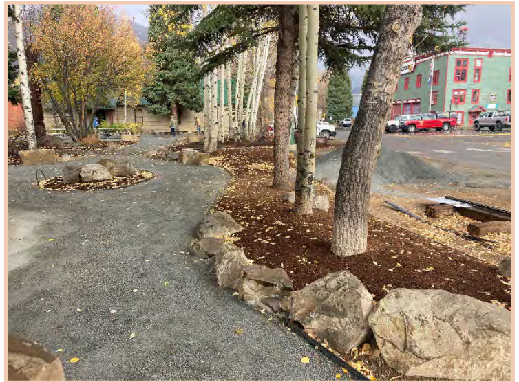
Totem Pole Park Renovation Project
