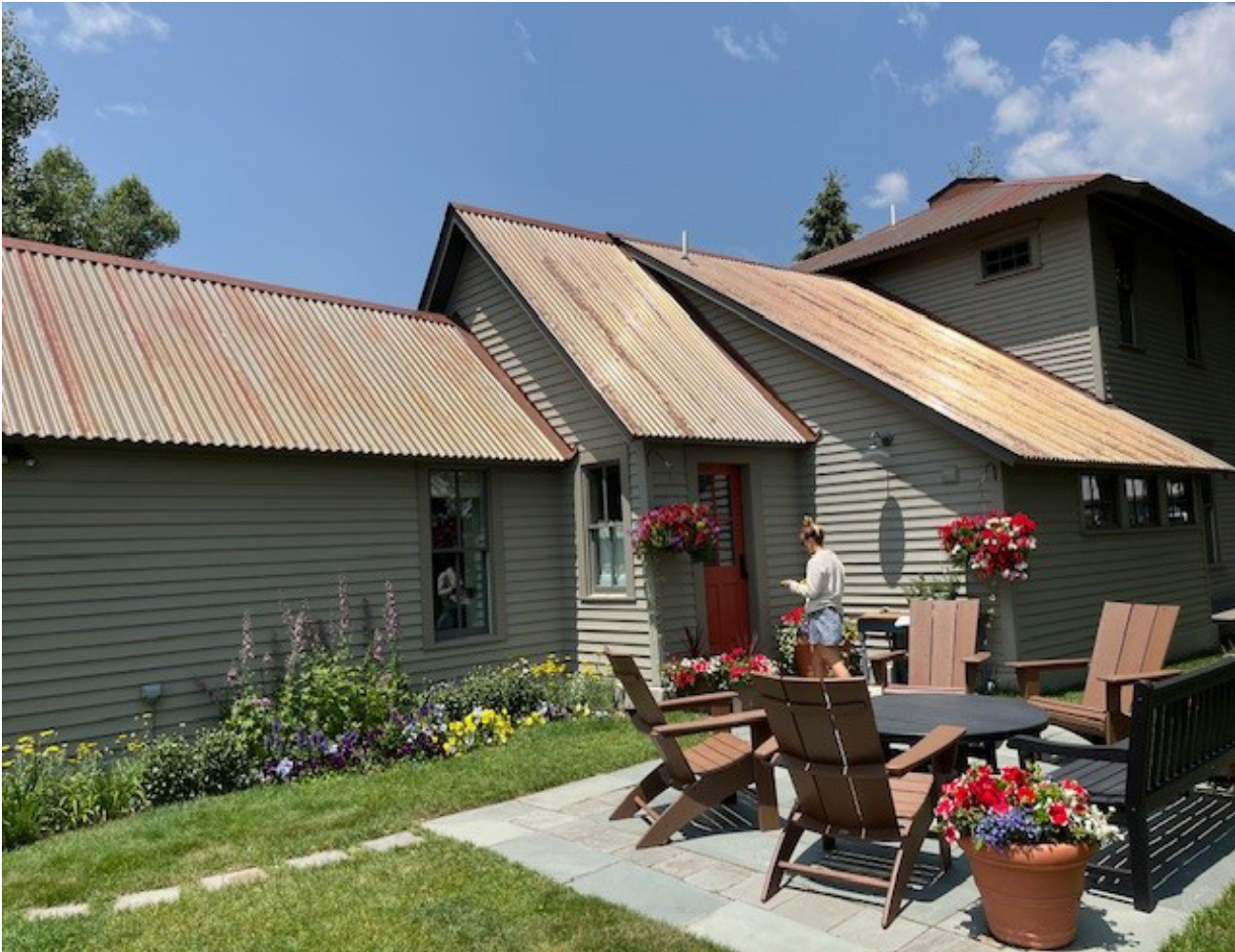
painted wood clapboards dimensions and color to match existing
