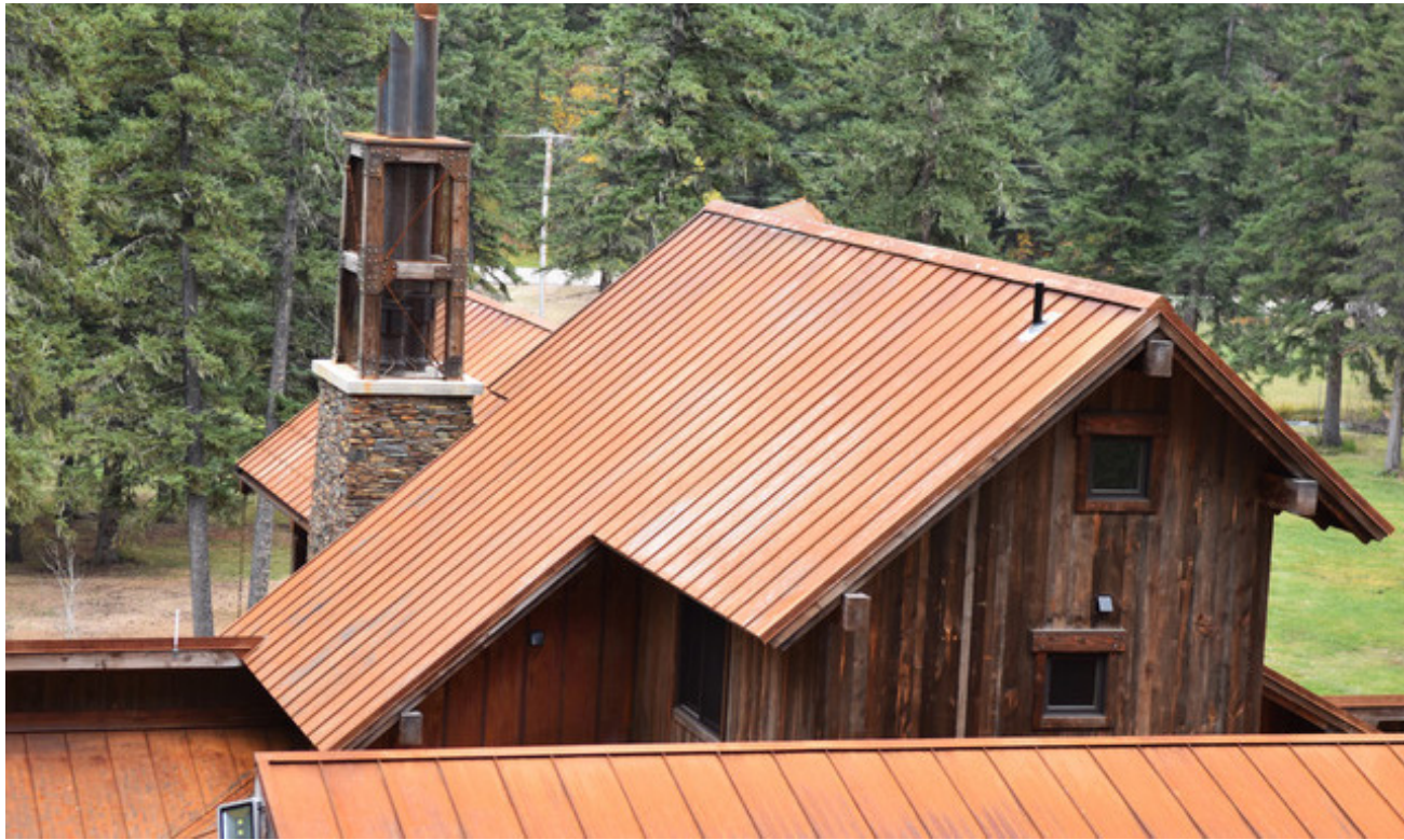
Proposed weathering steel standing seam
