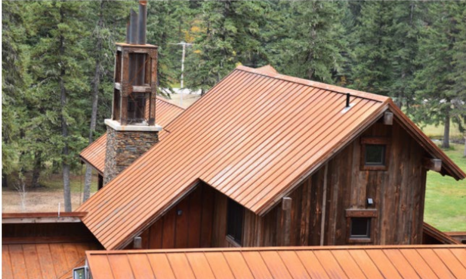
Proposed weathering steel standing seam
